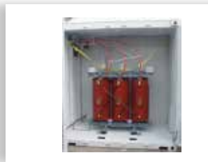
CTE MV Containerized Transformer Substation
