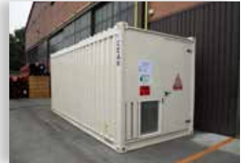
CT-PC – Containerized Power/Control Cabin
